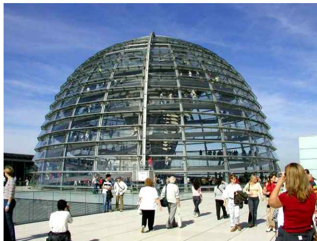
On the roof of the Reichstag
